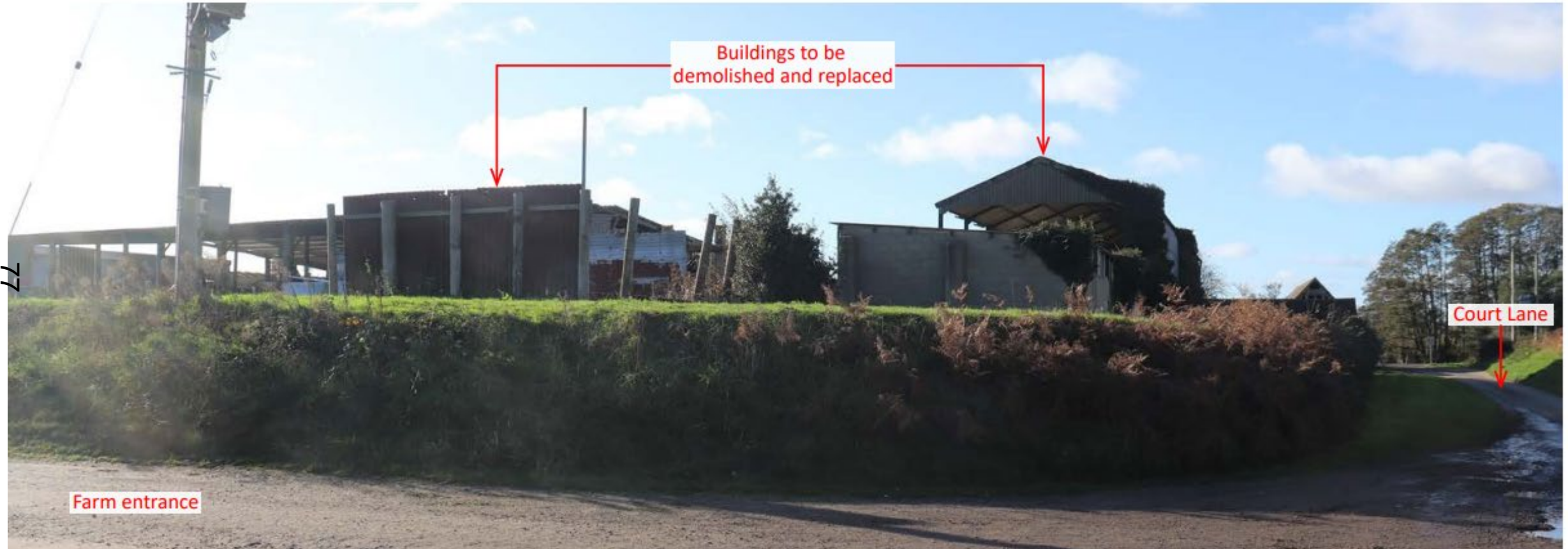
Existing buildings viewed from north east
